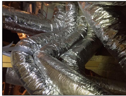
1.19 Picture 2 More excessive ductwork in the attic
