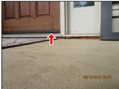
1.2 Picture 1 Worn out door fins on front door
