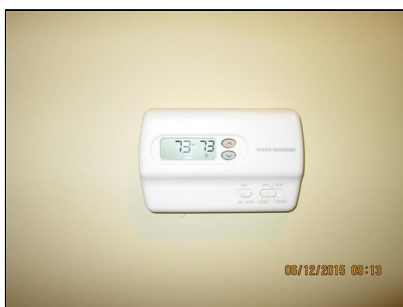
1.20 Picture 2 Basement system thermostat is not programmable
