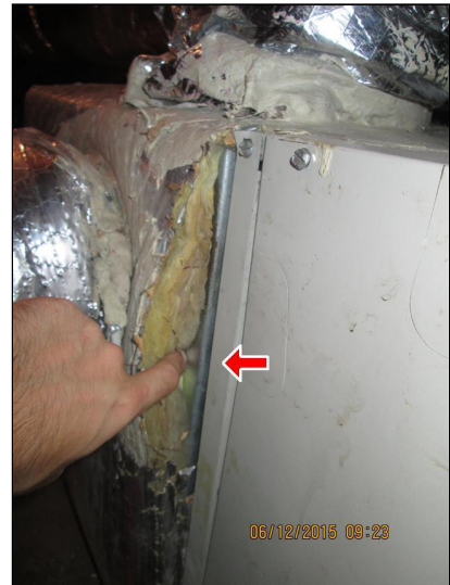
1.19 Picture 3 Insulation poorly attached to attic system plenum/air handler
