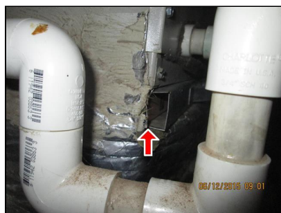
1.18 Picture 4 A poor fit for the basement system filter door
