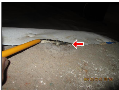
1.17 Picture 2 Poorly sealed vapor barrier, allowing moisture in crawlspace
