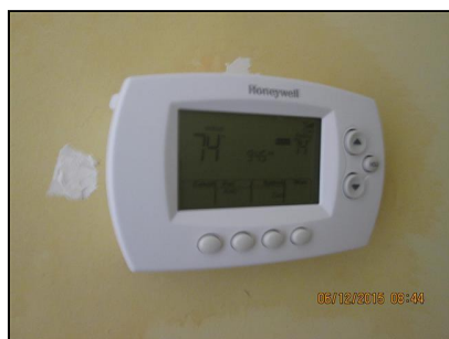
1.20 Picture 1 Programmable thermostat present for the main floor system. Great work!
