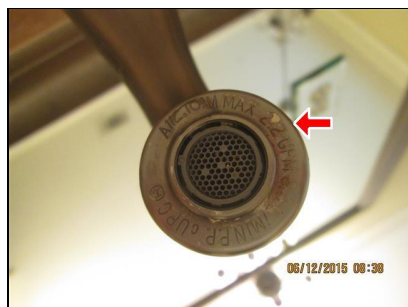
1.22 Picture 1 2.2gpm aerators throughout the home consume more hot water than low-flow aerators
