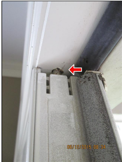
1.2 Picture 4 No strikeplate for double door deadbolt
