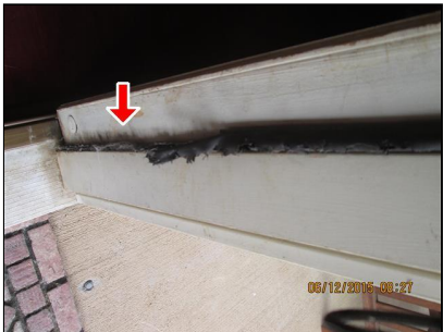
1.2 Picture 2 Front door weatherstripping is in very poor shape
