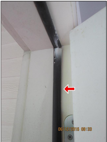
1.2 Picture 3 Kitchen double doors have compressed weatherstripping
