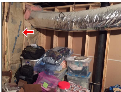
1.16 Picture 2 Batt insulation is an ineffective air barrier
