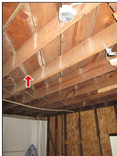
1.14 Picture 1 Zero subfloor insulation in unconditioned crawlspace
