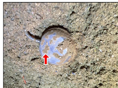
1.7 Picture 3 Cellulose attic insulation has melted to the can light
