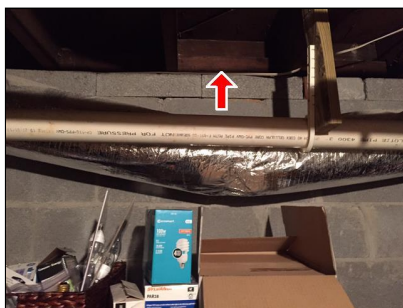
1.15 Picture 2 No insulation of rim joist
