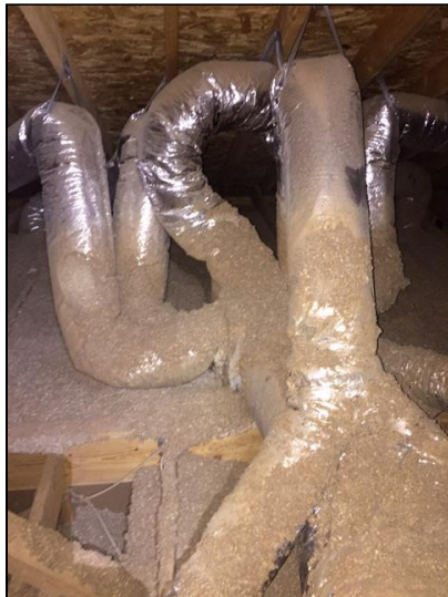
1.19 Picture 1 Excessive attic ductwork
