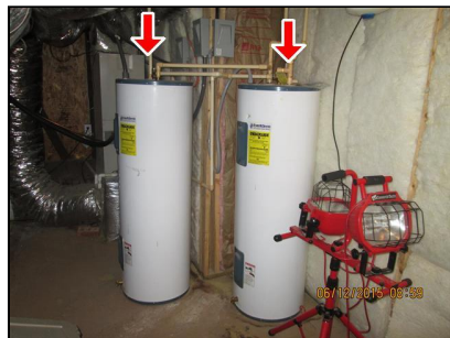
1.21 Picture 1 Water heaters in the unconditioned basement are uninsulated
