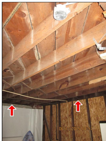
1.15 Picture 1 Zero rim joist insulation
