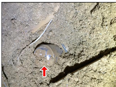
1.7 Picture 2 Insulation touching non-IC Rated can lights is a fire hazard
