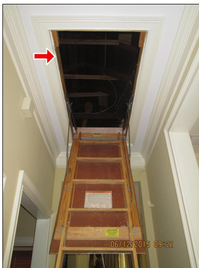
1.10 Picture 2 No air sealing measures present on attic access
