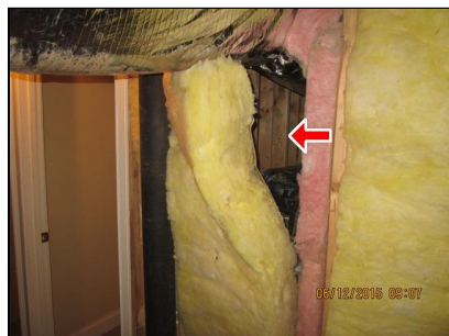
1.16 Picture 1 No air barrier present, meaning air can freely pass between unconditioned crawlspace and conditioned basement
